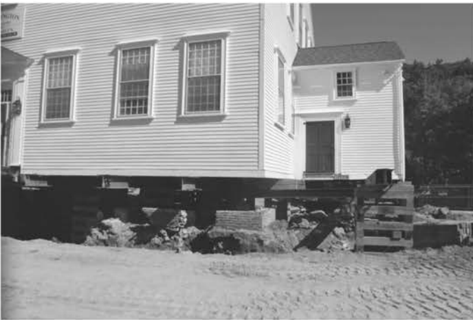
23 of these jacks were used to raise the Town Hall. It was estimated to weigh 200 tons.
