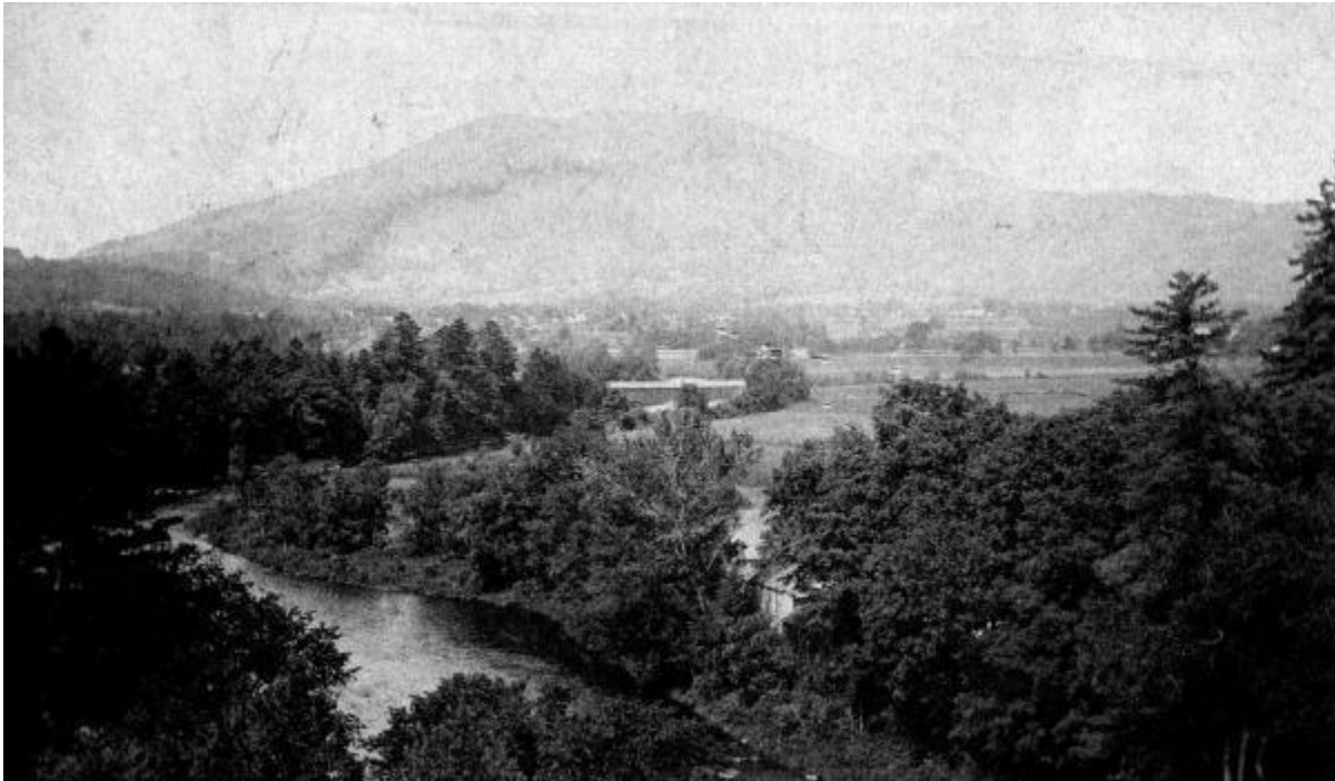
Lottery Bridge, across the Sugar River in West Claremont. The 2nd NH Turnpike terminated just north of this bridge where it joined an existing road, which ran long the Connecticut River. Photos of this bridge are hard to come by as it was replaced in 1892. The roof of the bridge is barely visible as a long white line in the center of the picture. Photo courtesy of Colin Sanborn from the Claremont Historical Society collection.
