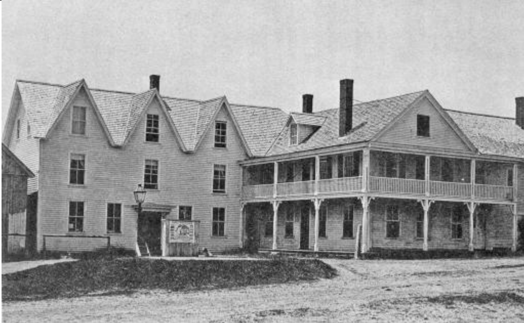
Store and residence of N. A. Lull & Sons, which was located slightly to the east of where the present general store now stands. It was also known as Davison's store when A. B. Davison ran it in the late 1880's. Picture from the 1886 "History of Washington, New Hampshire."
