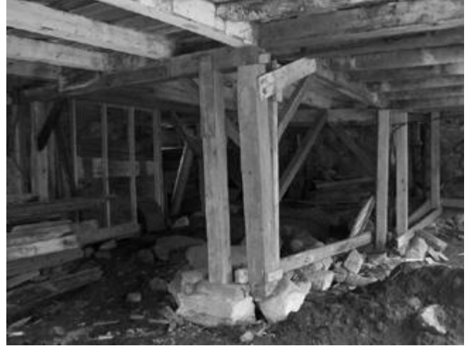
Basement excavation underway, showing old support beams and natural rock foundations
