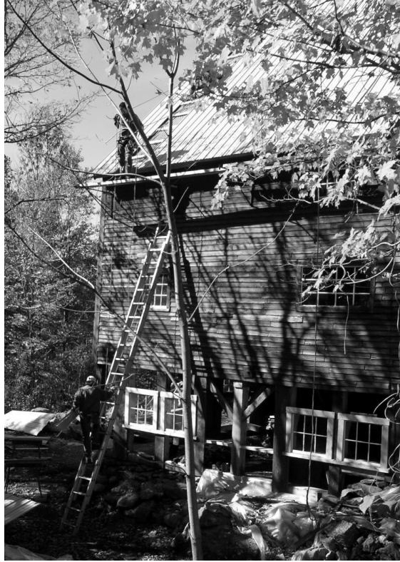
Workmen in fall -- even without color the beauty is evident.
